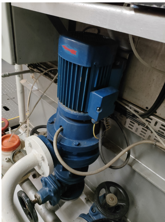
Figure 111: Sewage Discharge Treatment Pump
