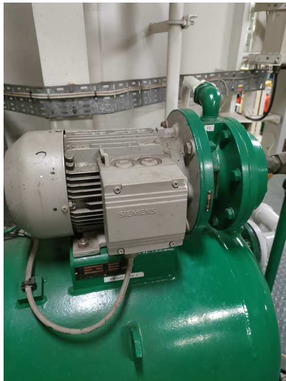
Figure 119: Vacuum Pump
