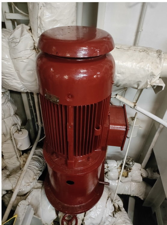
Figure 66: Fuel Oil transfer Pump
