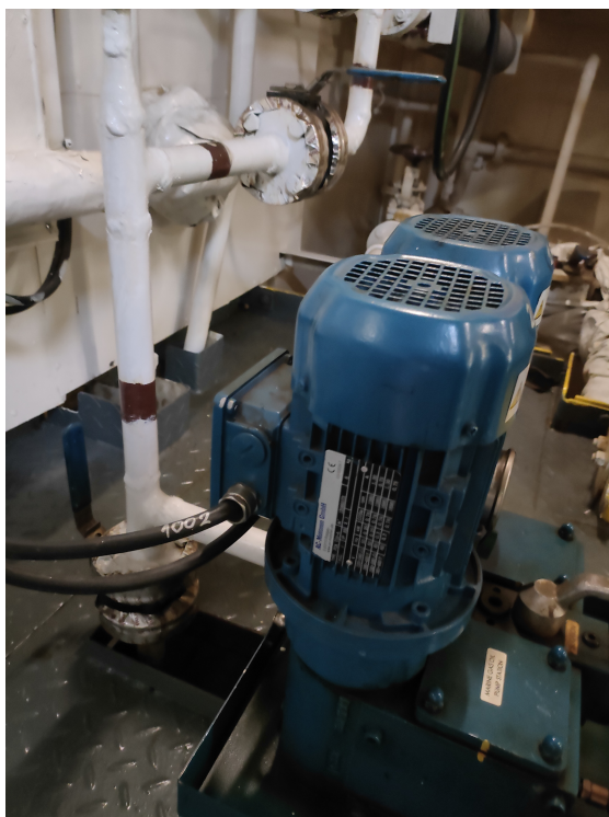
Figure 54: Feed Pump For Boiler
