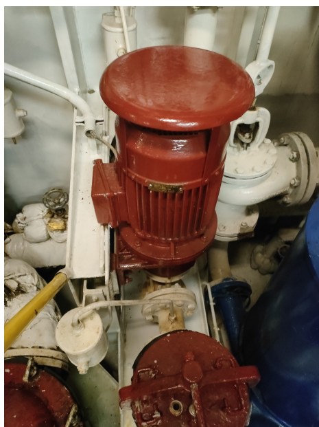
Figure 35: Diesel Oil Transfer Pump
