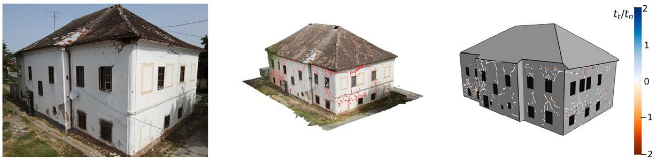
Figure 11: DADT for free-standing masonry buildings whose damage is mainly cracks—View 2 (buildings A to E from top-down). (a) Image view of damaged building. (b) 3D textured models of the buildings merged with spatial information of the cracks. (c) DADT of LOD3 + cracks characterized via kinematics.
