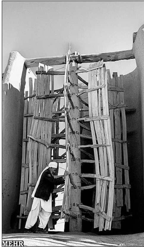
Figure 11. windmill in Nashtifan village, Iran, built with the traditional design, source: Mehr News Agency, Amir Ghaderi.
