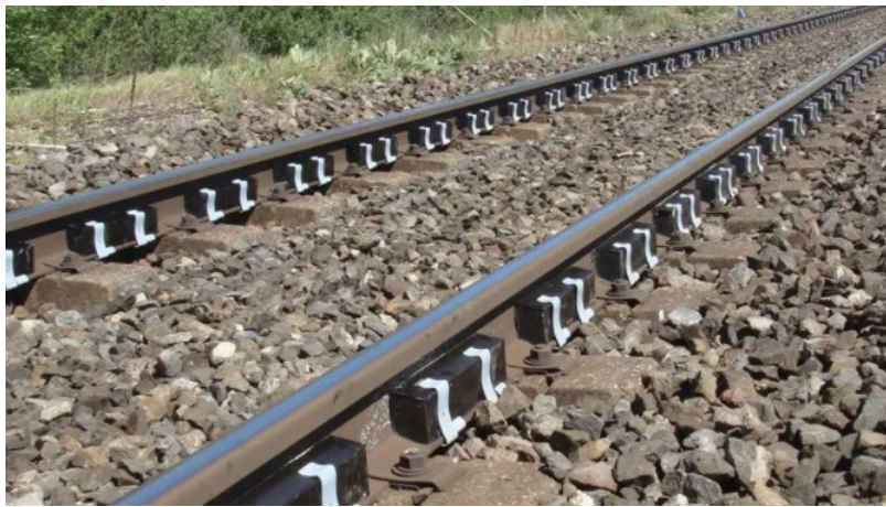
Figure 2.11 Rail vibration dampers.
