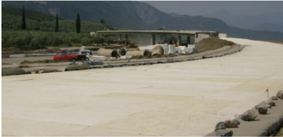
Figure 2.17 EPS application on Maliakos Gulf as highway embankment fill material.
