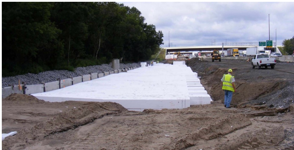
Figure 2.18 Widening of roads with the use of EPS geofoam.
