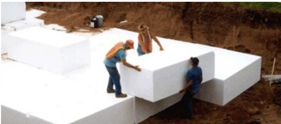
Figure 2.16 Implementation of EPS at the field with bare hands.
