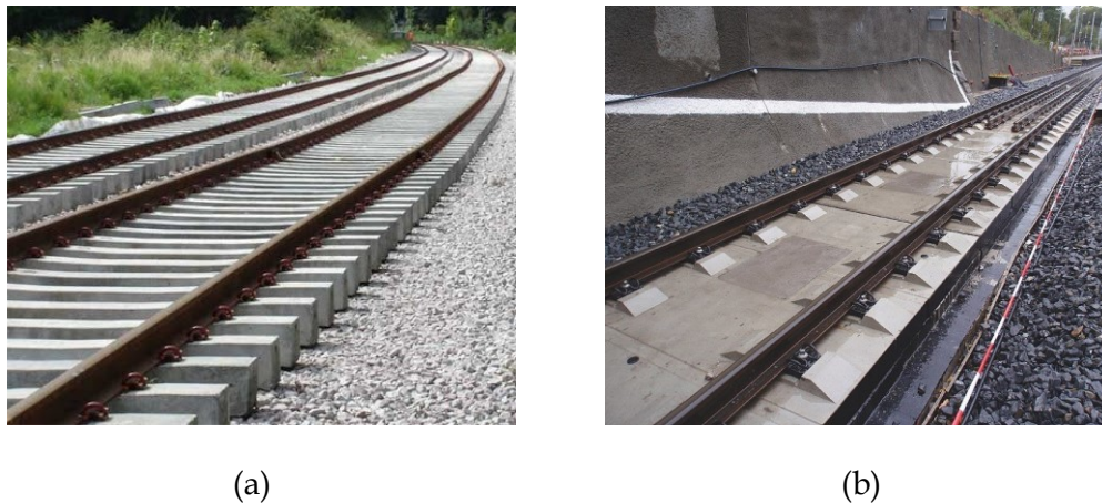
Figure 2.8 (a) Ballasted track, (b) ballastless track.
