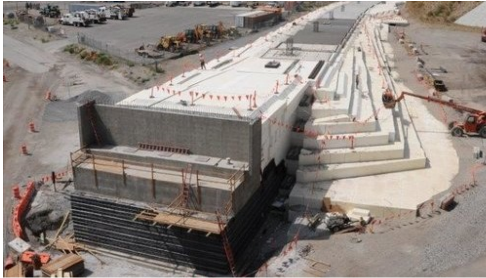
Figure 2.20 EPS Geofoam Embankment, UTA light-rail system, West Valley Line.
