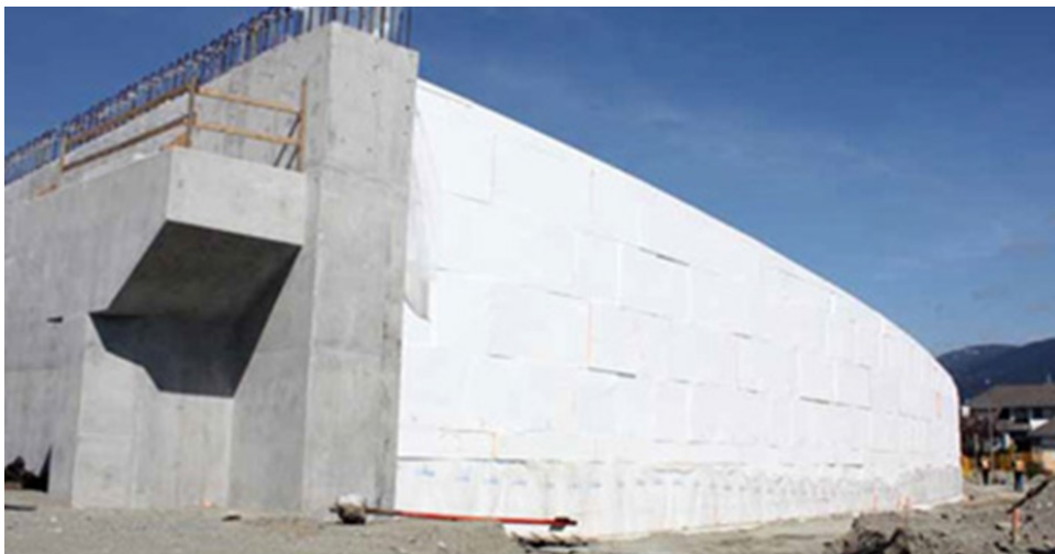
Figure 2. 19 EPS as bridge abutment.
