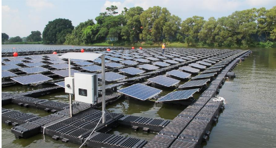
Figure 2: HPDE modules for Photov. Panels support at 500kW FPV Plant in Singapore.
