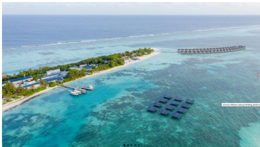
Figure 6: Swimsol 191kW coastal FPV Plant, South Ari Atoll, Maldives.
