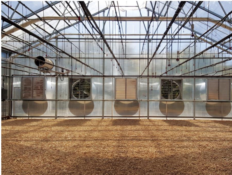
Figure 1.16: Fans arrays of dynamic greenhouse ventilation system [31].
