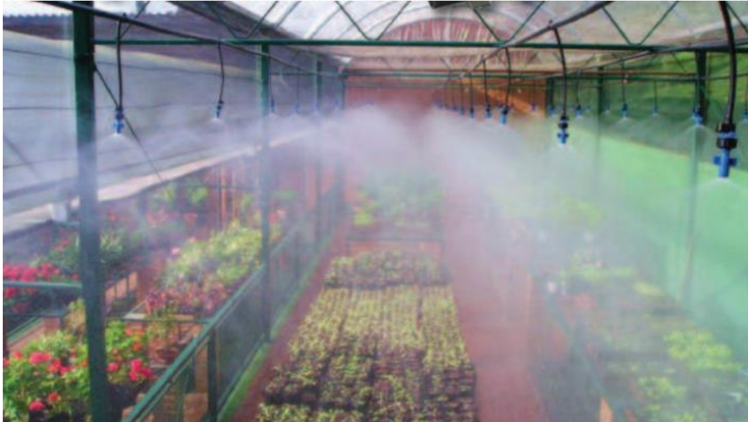
Figure 1.17: Sprinkler cooling system [32].
