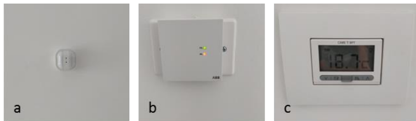
Figure 21: a) Presence sensor, b) Air quality sensor, c) HVAC thermostat.
