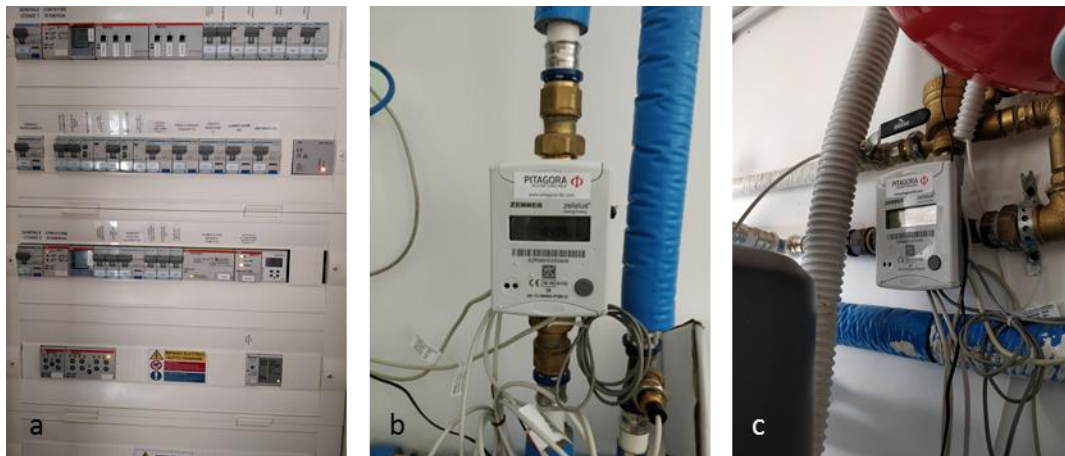
Figure 22: a) Electricity metering, b) Heat pump energy meter, c) DHW meter.
