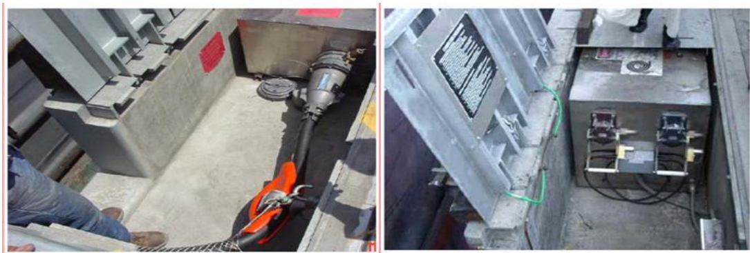
Figure 2.8 Connection box with one connector on the left and with two connectors on the right.
