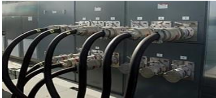
Figure 2.7 Cables for Cold Ironing Connection [6]
