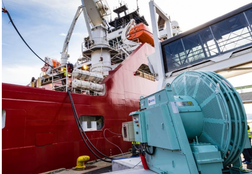
Figure 2.11 AMP Reel of CAVOTEC [7]
