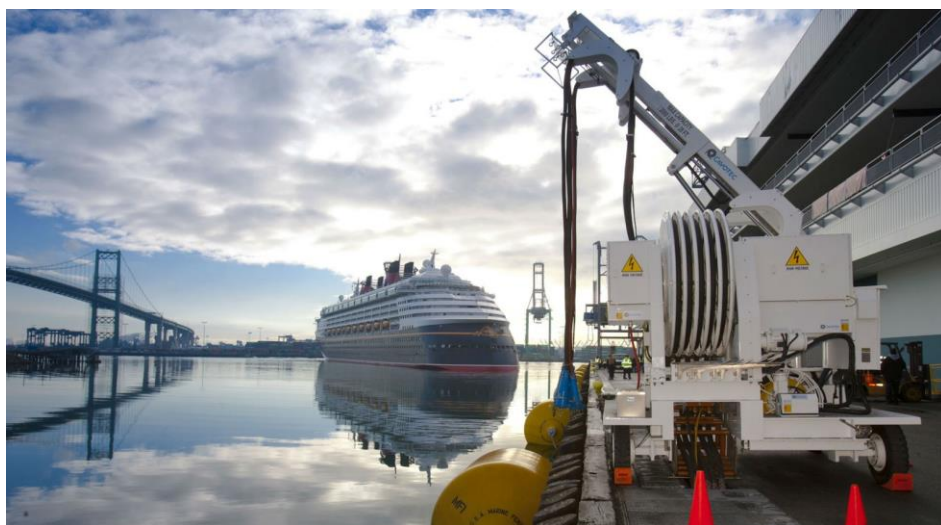
Figure 2.1 Cold-Ironing equipment in port of Los Angeles [1]
