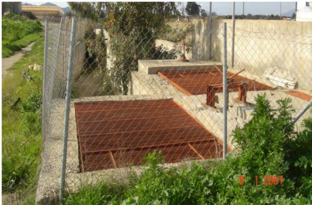
Figure 3. Transmission channel of water for the recharge of the Messara aquifer. (Bouloukakis , 2007)
