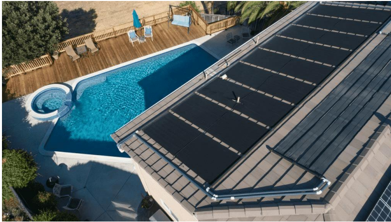
Figure 1.13: Unglazed Solar collector [18]
