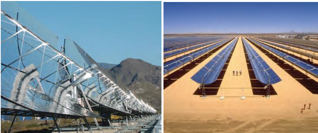
Figure 1.22: Parabolic trough collectors systems [1]
