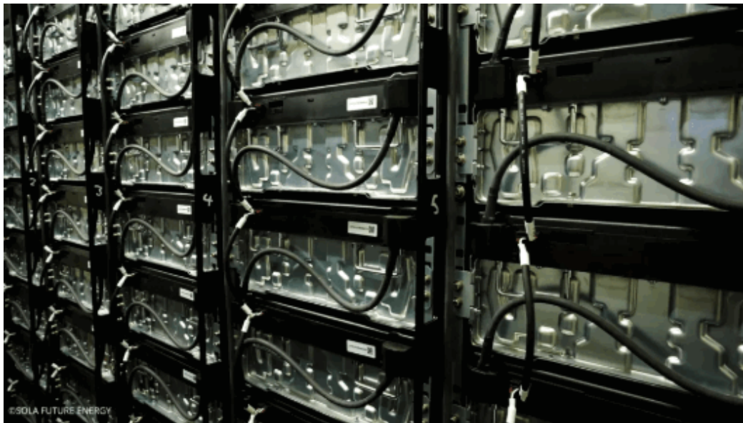
Lithium-ion batteries store excess solar PV at Robben Island Microgrid
