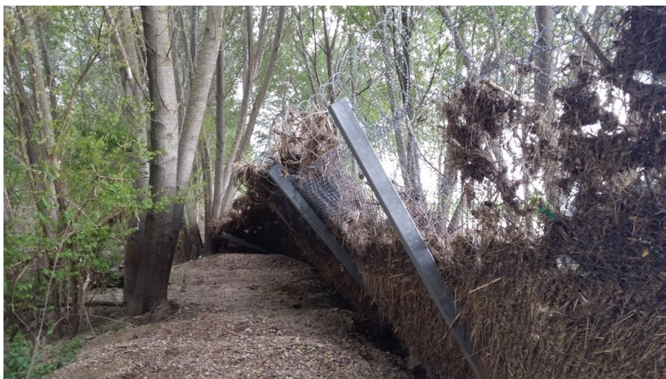
Image 15: Technical fence preventer after the flood damage
