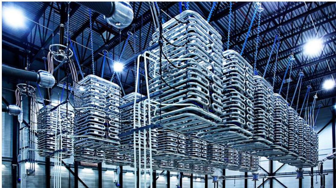
Figure 2.7: Valve hall of 500 kV, 700 MW Skagerrak 4 Modular Multilevel Converter (MMC) (ABB, 2016)
