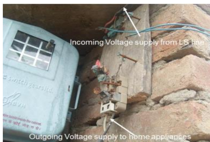
Figure 2.5 Method of stealing electricity.
