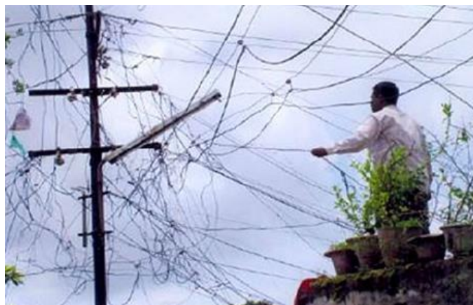
Figure 2.3 Method of stealing electricity.
