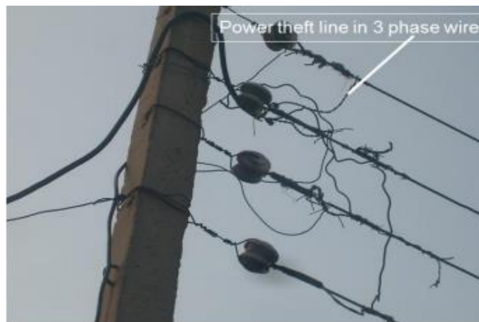
Figure 2.1 Method of stealing electricity.
