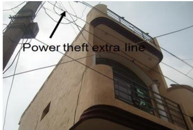
Figure 2.2 Method of stealing electricity.
