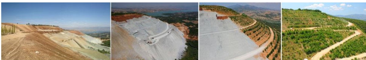
Figure 2.6: Procedure of asbestos mine rehabilitation
