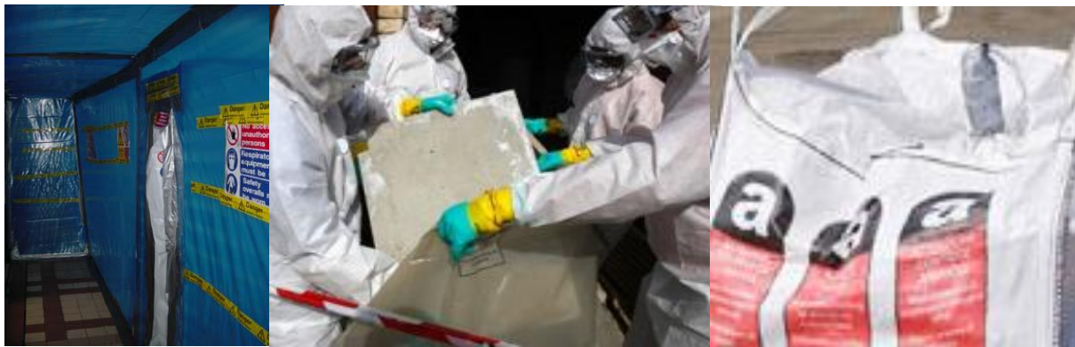
Figure 2.7: Procedure of asbestos containing materials dismantling and packaging
