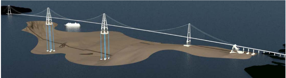
c) Suspension bridge with floating pylons (towers)
