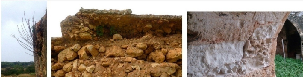
Figure 4. External view of the north masonry of [D] and the developed tree (left). Internal layer of eastern collapsed façade and cement mortar covering (middle). Alteration of stone surface of the pillars of [E] chamber and material loss (right).
