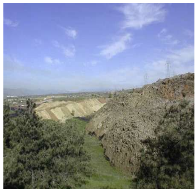
Figure 4.2: The failure moving face plus the first berm under-construction [Steiakakis et al., 2009].
