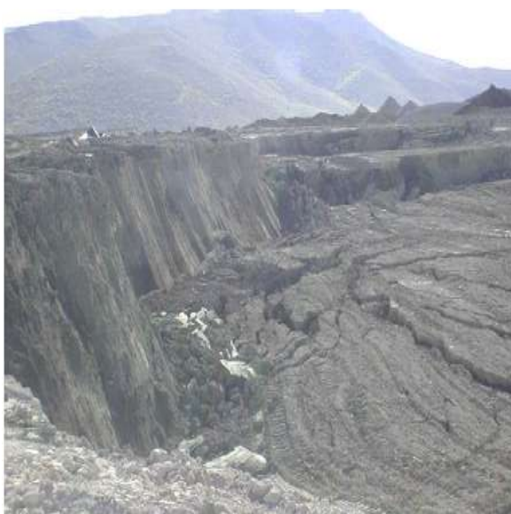
Figure 4.1: The crest of the dump failure [Steiakakis et al., 2009].
