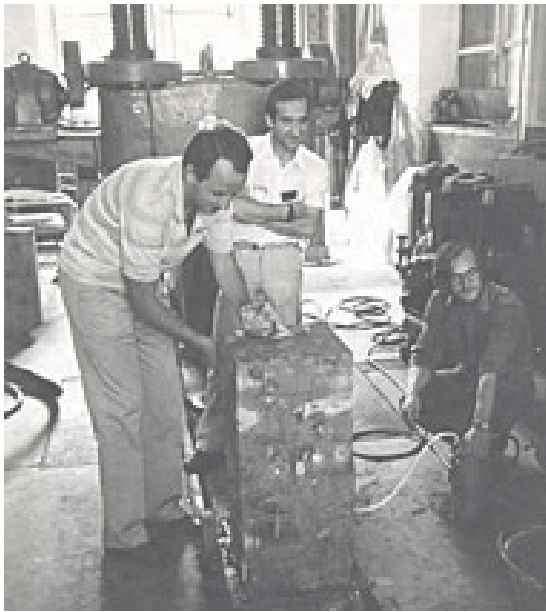
εικ. 25: Further testing at the University of Rome in 1982. An experimental wall, partially crushed under a press, is consolidated by grout injection.
