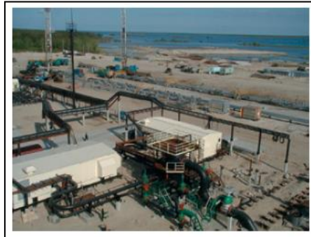
Figure 38: Installation of 4 helicoaxial MPPs of Sulzer Company, in Priobskoye oilfield in Siberia [57].
