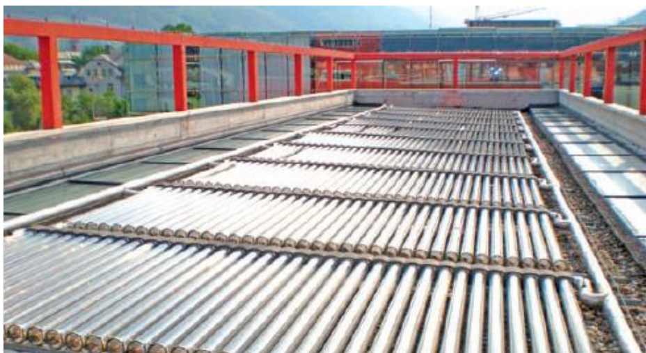
Figure 22: Vacuum tubes collectors on the roof of EURAC, Bolzano [41]
