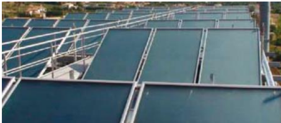
Figure 20: Selective flat plate collectors in CRES, Athens, Greece [10]
