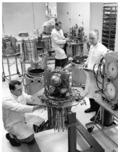
Fuel cell powerplants, to provide on-board electricity for the Apollo command and service modules (and the by-product: drinkable water), being developed by Pratt & Whitney Aircraft, May 18 1964.
