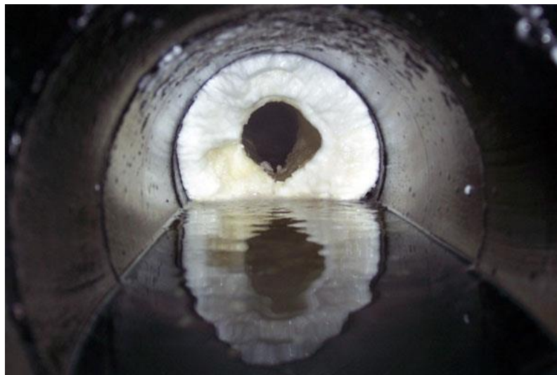
Figure 3: Flow restriction due to hydrate formation and agglomeration on the pipeline wall
