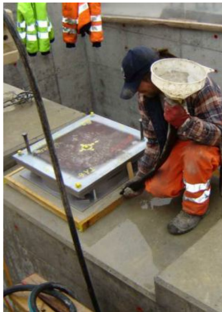
FIGURE 2.13: Construction and Installation of the Mortar Bed using the free flow mortar
