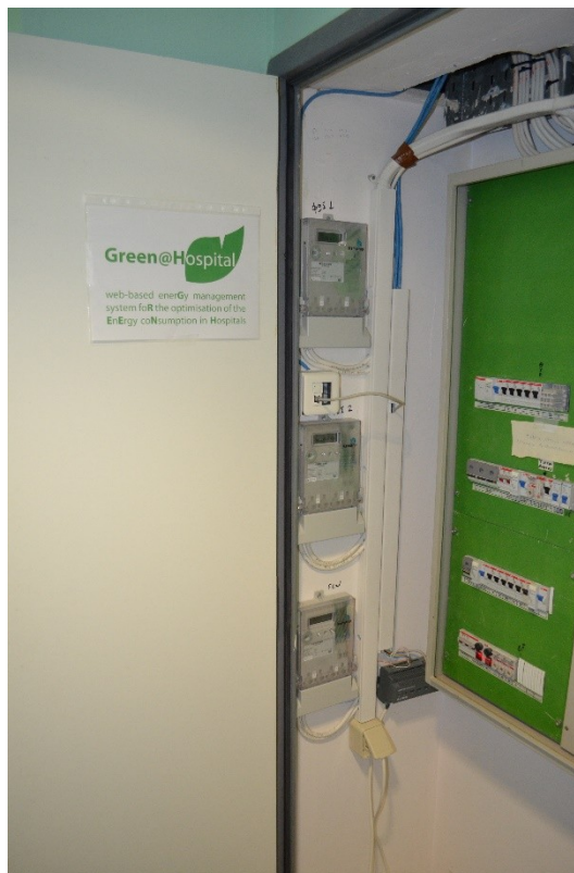
Figure 7- 2: The installed controller in each room of the paediatric department
