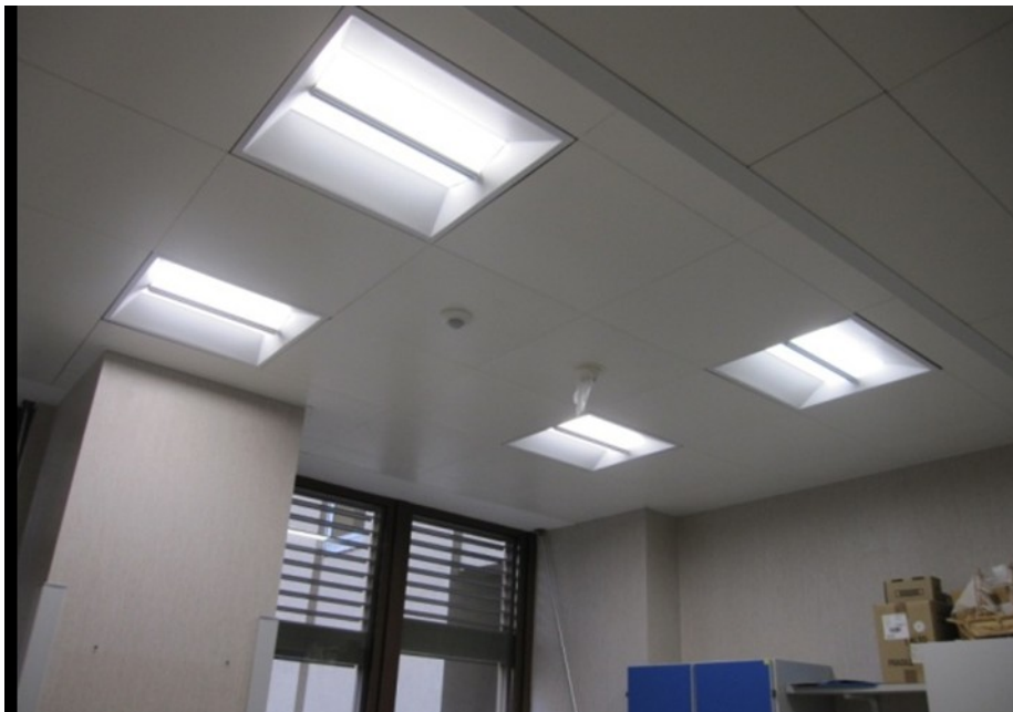
Figure 7- 7: Update of light infrastructure using LED lights and presence detector
