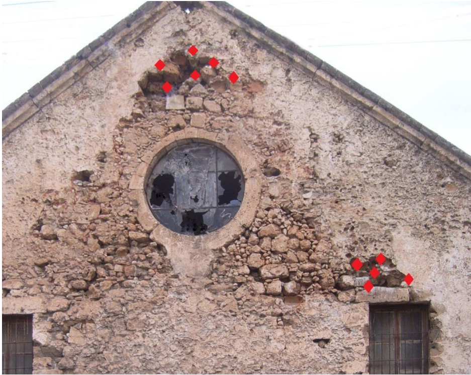
Figure 4.10 An example of the measurements we acquired of some of the damages. We focused on measuring their outline and their depth.
