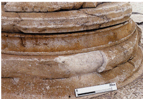
Image 4. Decay observed accompanied By ablation of parts of the stone Consequent upon mechanical reasons
