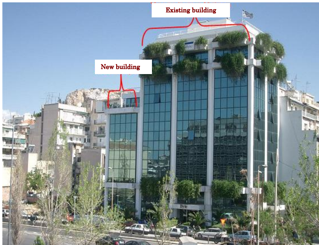
Figure 4-1: The Building of BYTE
